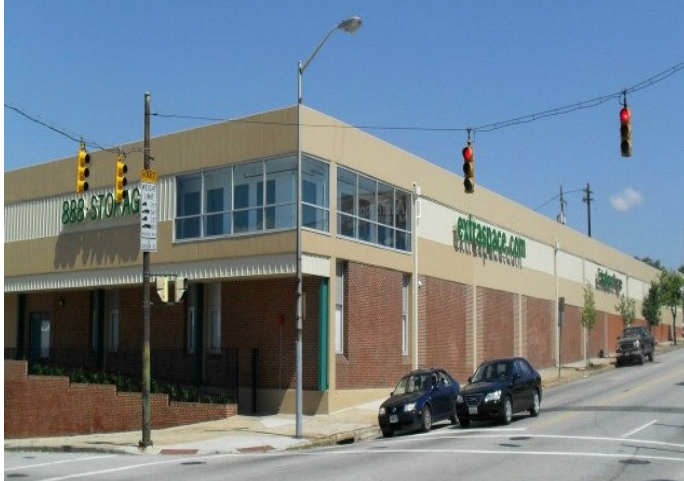
Extra Space Storage Howard Street Property
