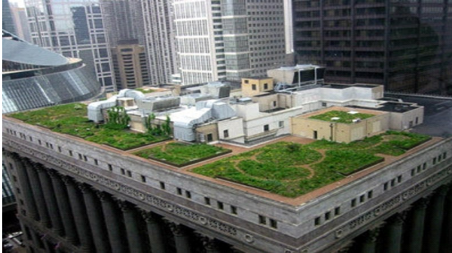
Chicago City Hall Green Roof
