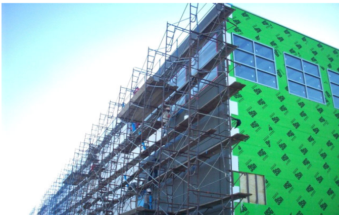
Construction Of Four Story Storage Building At Pasadena
